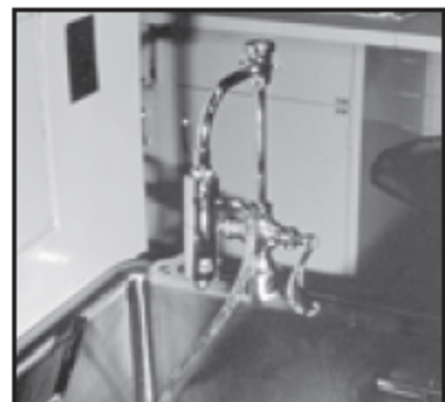
FIGURE 17. Atmospheric vacuum breaker in plumbing supply system.
